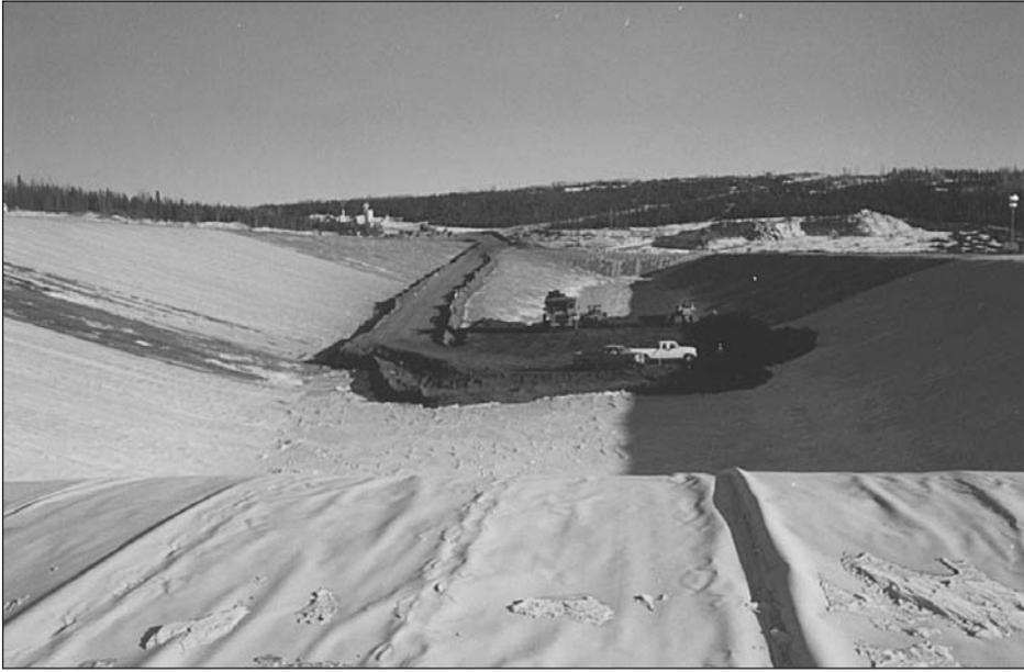
**FIGURE 1 Ore placement at in-heap solution storage facility (Alaska heap leach project)**
