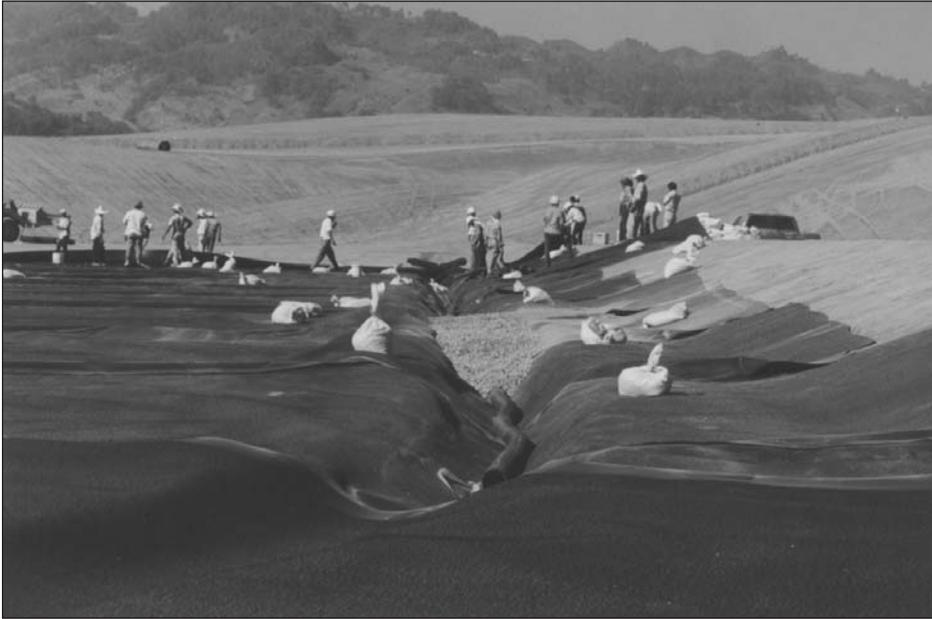
**FIGURE 3 Substantial regrading, use of textured liner and intermediate anchor trenches at a steep leach pad site in Central America**
