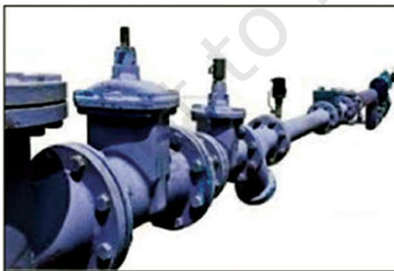
Fig. 5.27: Flanged joints
